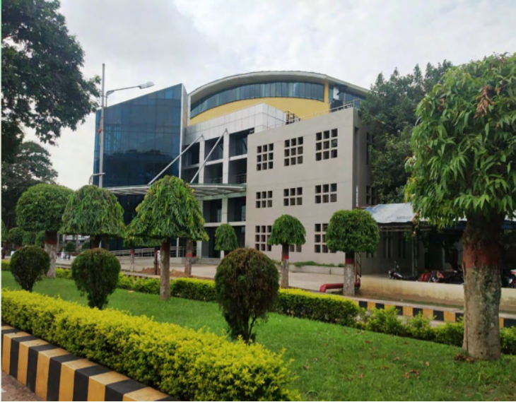
New Auditorium Hall
